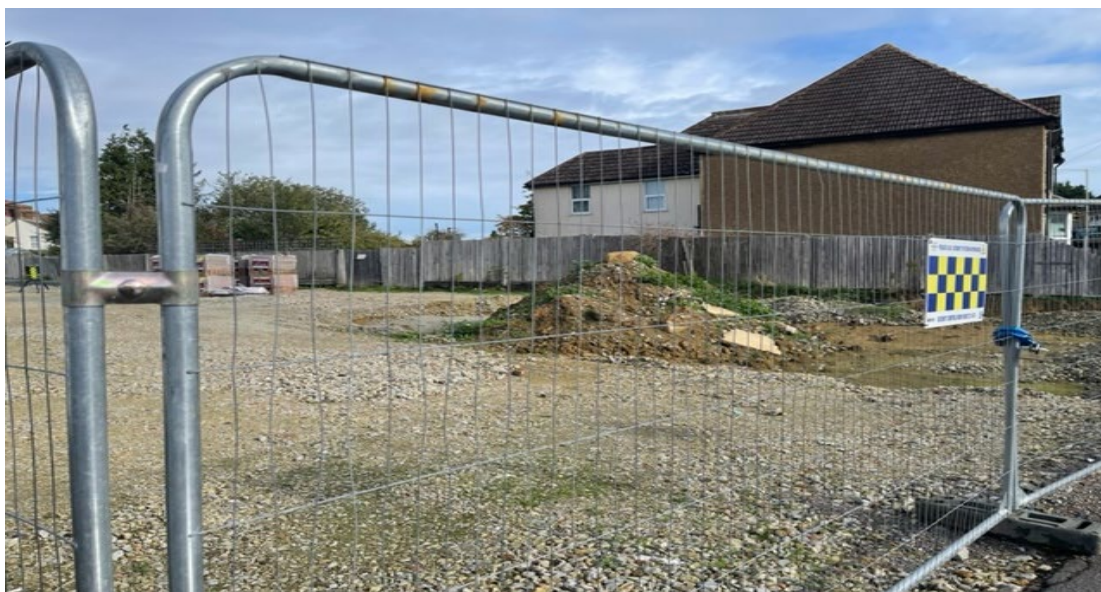
Figure 3: Photo showing the flank elevation of the dwelling. The adjacent car park (under construction) in the foreground
